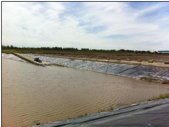
Figure 3 – Snow disposal detention pond for treating melt water
