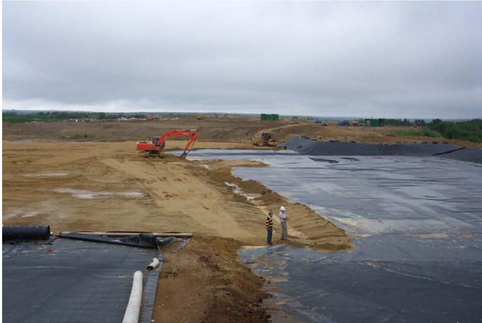
**Figure 6: Synthetic liner at the landfill in the north of Sakhalin (photo by A. Chaikine)**
