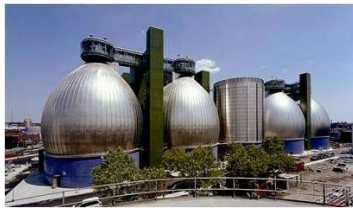
Wastewater treatment plant digester
