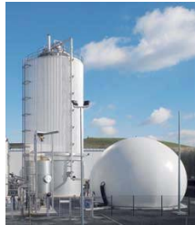
Wet High-Solids or Dry Pumpable
