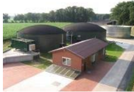
Wet Low-Solids e.g. Dairy
